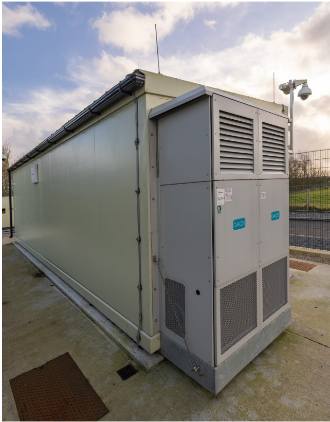
Figure 6. Air conditioning Unit
