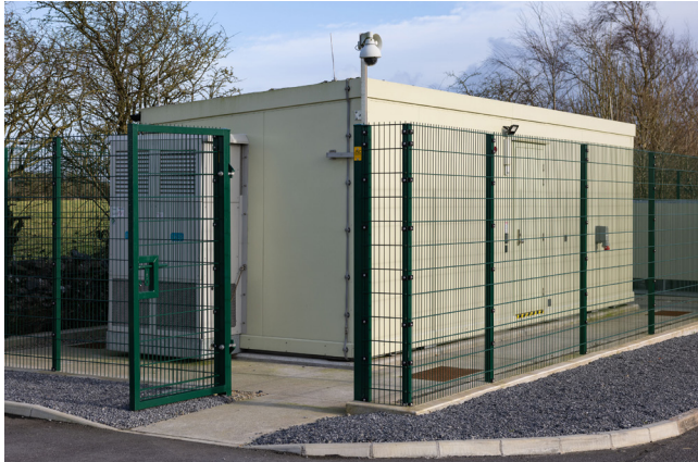
Figure 1. Gaybrook Co-location Facility
